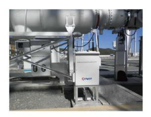
PDMonitorU utilizes UHF, HFCT, and AE Sensors to monitor, analyze, and diagnose the PD signals emitted from multiple high voltage electrical equipment.
